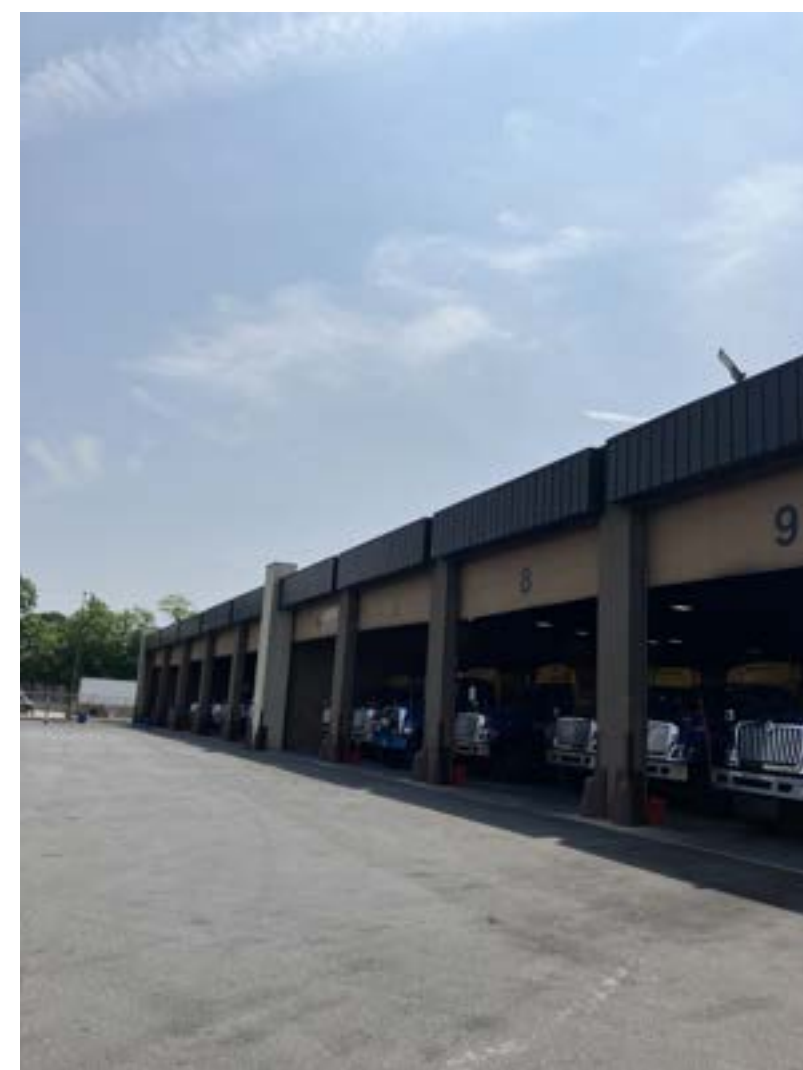
EXISTING BUILDING ELEVATION - YARD SIDE NEEDS NEW INSULATED GARAGE ROLL-UP DOORS.
