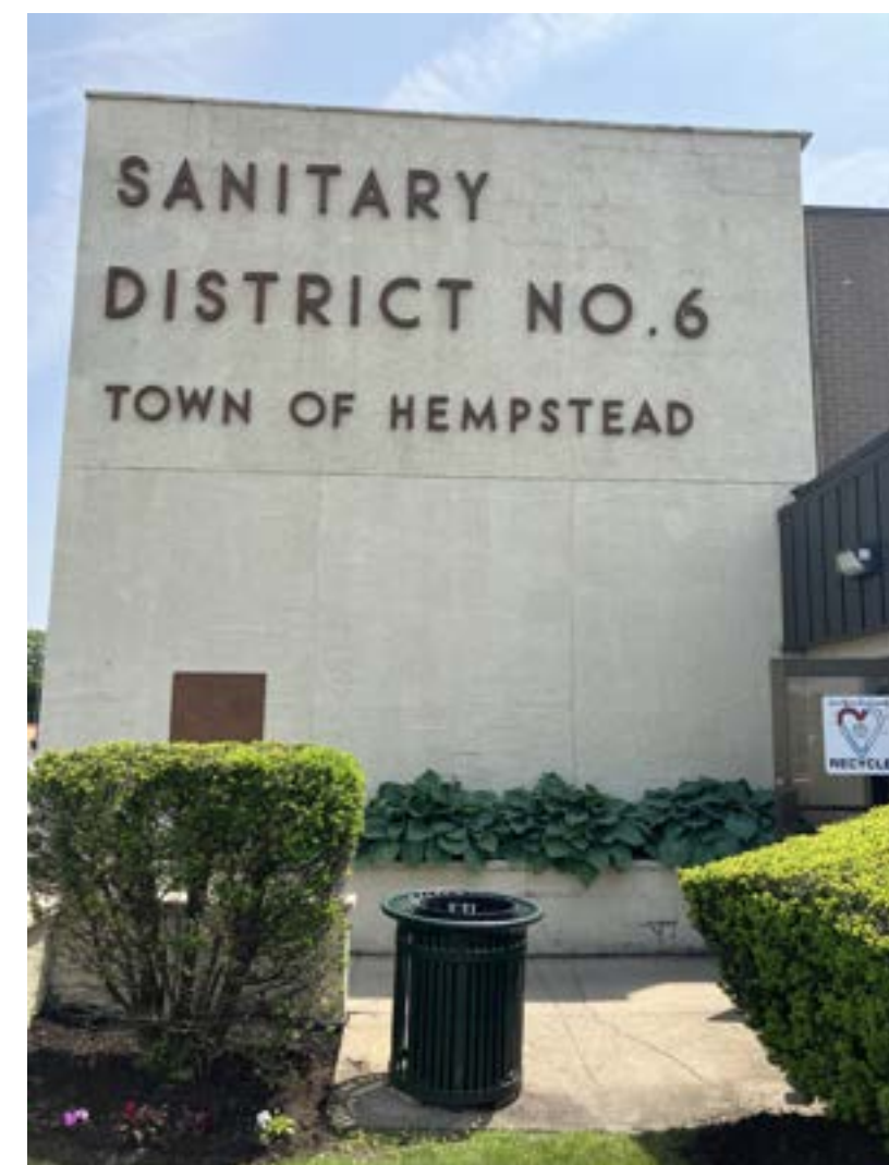
EXISTING FRONT ENTRANCE.
