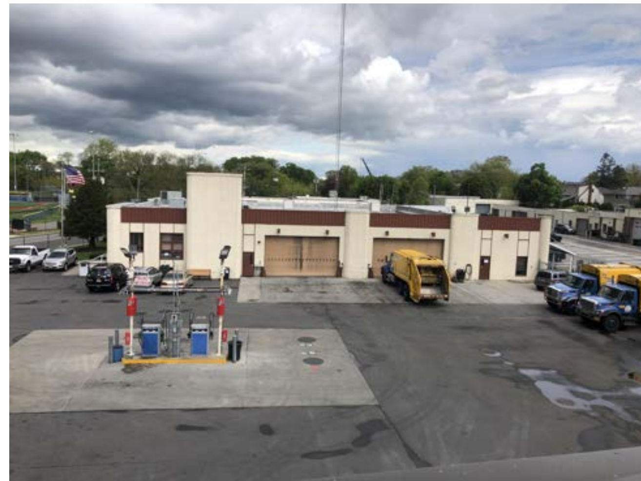
OVERALL EXISTING BUILDING ELEVATION - YARD SIDE.
